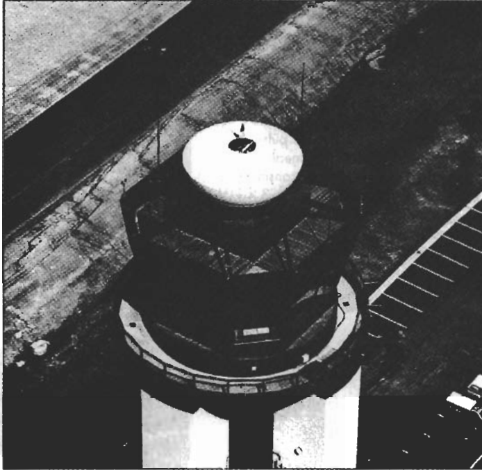
Figure 1.7 This ASDE-3 airport surface detection equipment is shown located on the control tower at the Pittsburgh International Airport. It produces a high-resolution ground map of the airport so as to monitor and expedite the movement of airport vehicle traffic and taxiing aircraft. This K_u -band radar operates from 15.7 to 17.7 GHz with a peak power of 3 kW, 40 ns pulse width, and 16 kHz pulse repetition frequency. The antenna and its rotodome rotate together at 60 rpm. The antenna gain is 44 dB, the azimuth beamwidth is 0.25^\circ (a very narrow beamwidth for a radar), and its elevation beamwidth is 1.6^\circ . It radiates circular polarization and has pulse-to-pulse frequency agility over 16 pulses, both of which help to increase the detectability of aircraft and vehicles in the rain. The display range is from 600 to 7300 m. The hole seen at the top of the rotodome in this figure is an access hatch that is not usually open. (It was open when this picture was made to allow a surveying instrument to be used for precisely locating the antenna.) Four lightning rods are shown around the rotodome.
